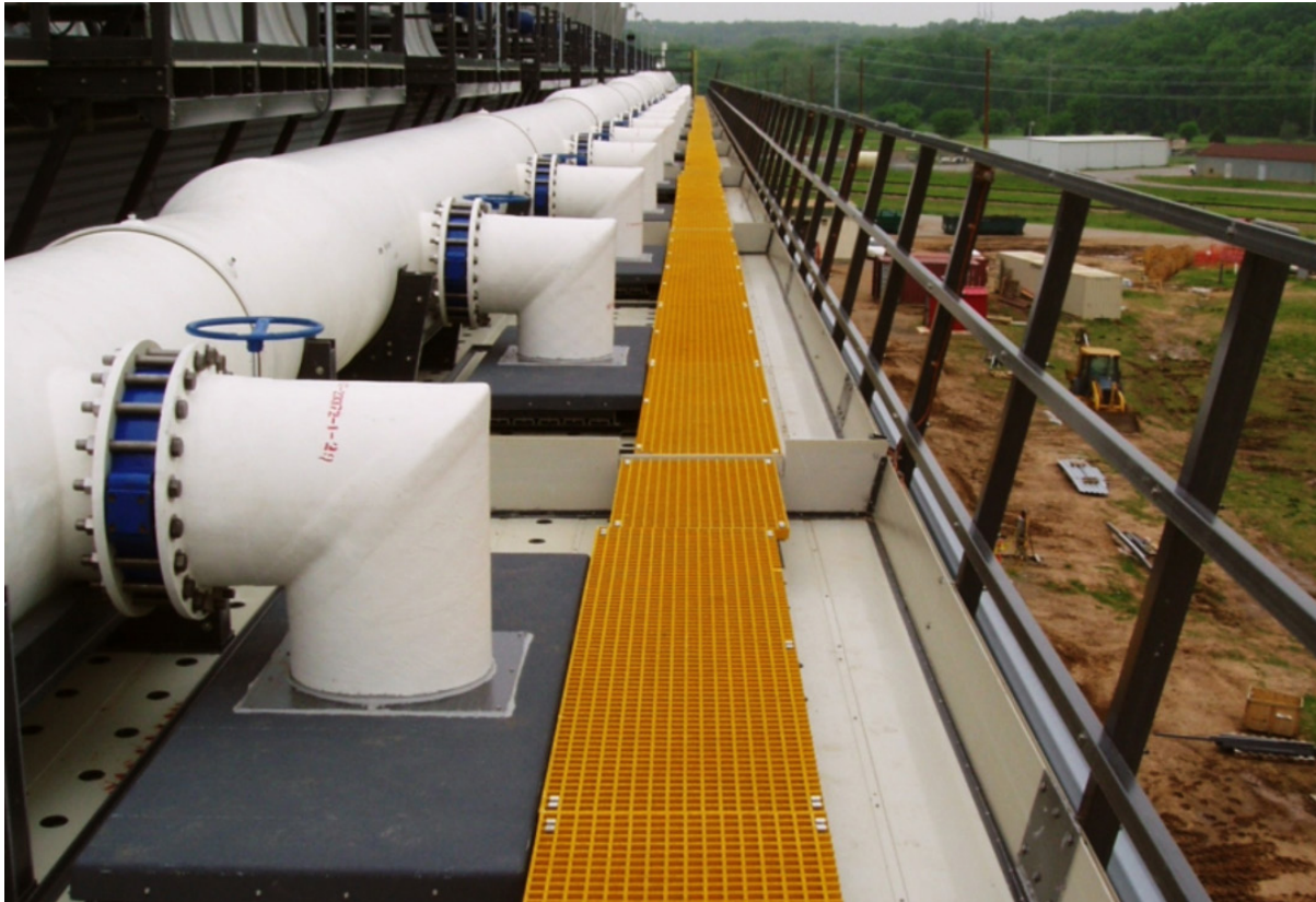
Post-Reconstruction Showing FRP Structural Enhancements
