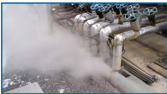
Leaking valves
