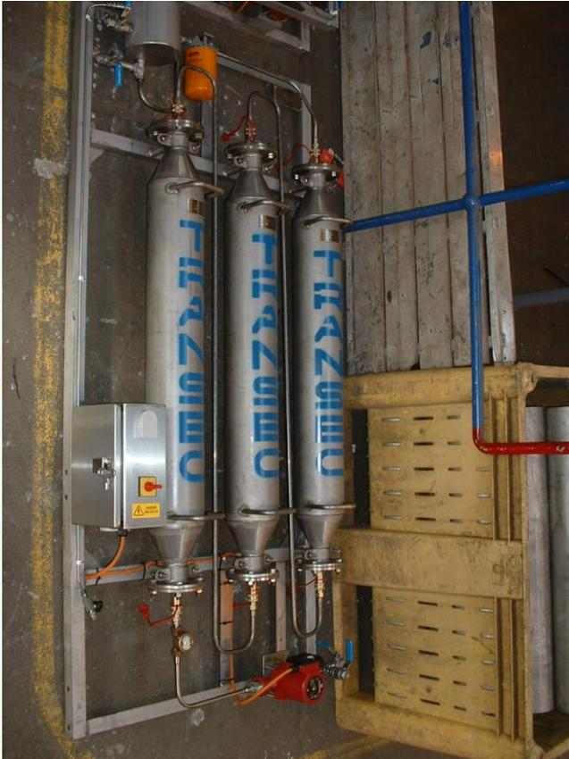
The picture shows the CL3AM monitoring enclosure in stainless steel, rated at IP65 with electrical isolator, mounted on the TRANSEC frame. The two MMT162 probe cables are terminated within the enclosure, from where the SCADA and alarm signals can be taken. The local LCD display is housed within the cabinet
