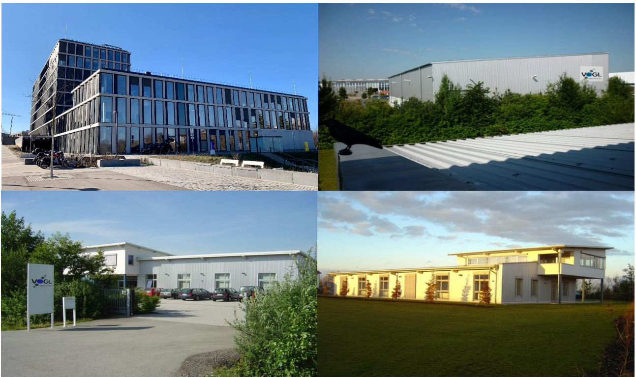
Figure 1: Research&Development (top left), High voltage test field (top right), Head office (bottom)
