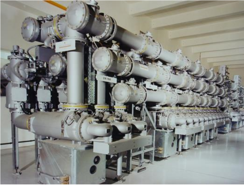
Figure 7: High voltage switchgear
