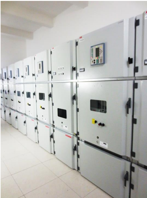
Figure 8: Medium voltage switchgear
